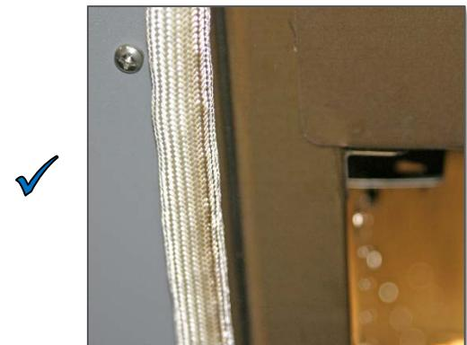
**Figure 9: Chamber Gasket Aligned**
